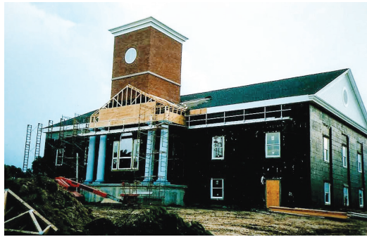
Construction progress of the new church
